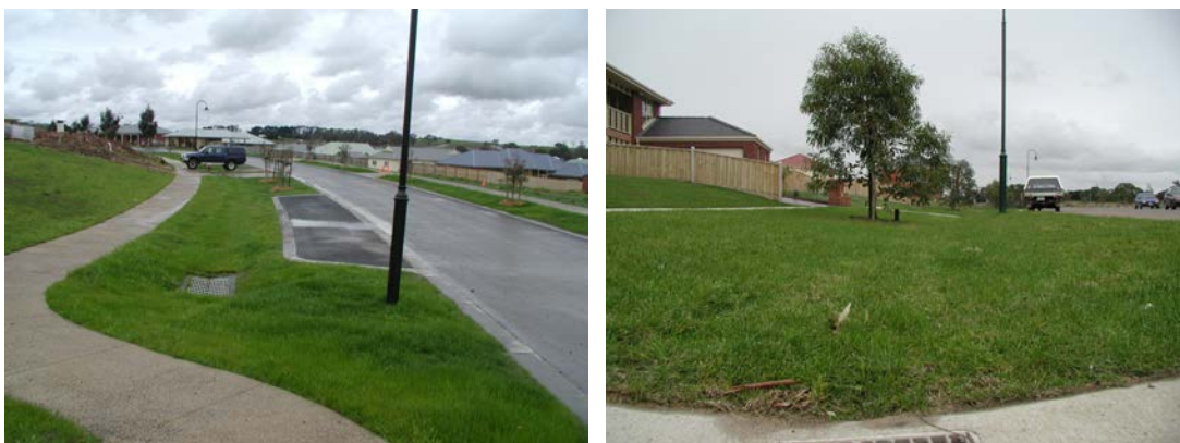
Figure 7.17. Similar buffer swale system for conveying runoff
