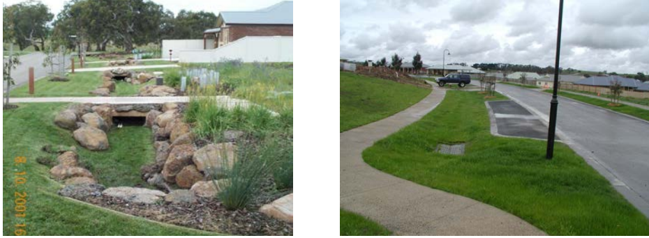
Figure 7.3. Elevated and at-grade driveway crossings across swales
