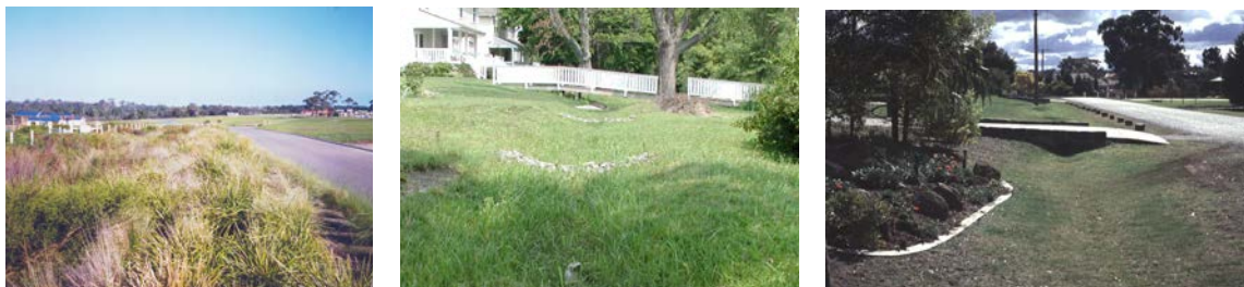
Figure 7.2. Swale systems: heavily vegetated, use of check dams, grass swale with elevated crossings
