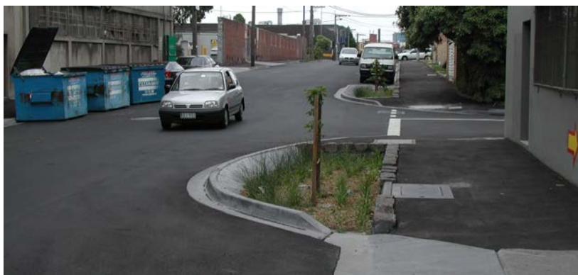
Figure 5.7. Retrofitted Bioretention System in a street
