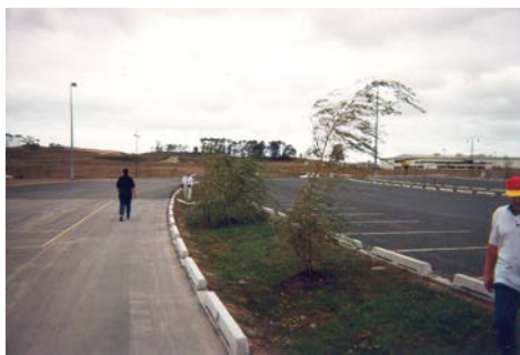
Figure 4.9. Photograph of kerbs with breaks to distribute inflows
