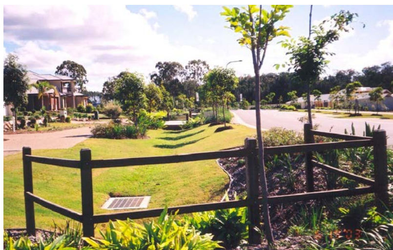
Figure 4.12. Photograph of bioretention swale
