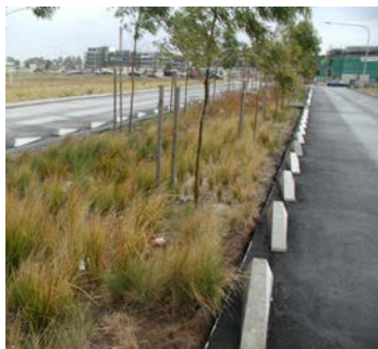
Figure 4.9. Photograph of kerbs with breaks to distribute inflows
