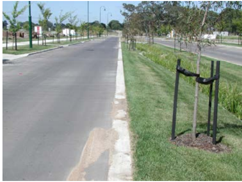
Figure 4.8. Photograph of flush kerb without setdown, edge detail showing setdown
