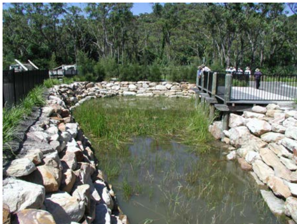
Figure 3.5. Illustration of Hard Edge Treatment for Open Waterbodies (GbLA, 2004)
