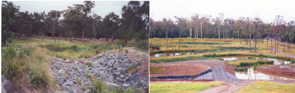
Figure 3.8. Overflow Structure of a Sedimentation Basin
