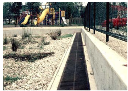
Infiltration systems are best suited to sandy soils with deep groundwater
