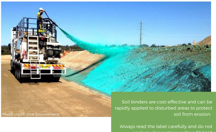
apply to slopes steeper than 3:1 (H:V)
