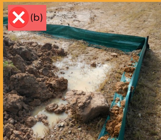
Well installed sediment fences (a) work effectively to pond runoff, allowing sediment to settle out via gravity, while poorly installed sediment fences (b) - where the fabric has not been correctly buried - do little to prevent sediment moving off-site. Images from TOPO Pty. Ltd.
