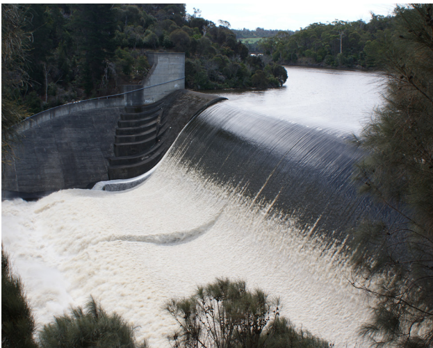
Above: Trevallyn Dam 'on-spill', with flows heading towards Cataract Gorge.
