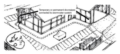
**2. Early drainage connection.** Connect downpipes and other drainage to the stormwater system as soon as the roof is on and / or other impervious surfaces are constructed, such as driveways, parking areas, or the building slab. Temporary flexible downpipes can be useful until permanent pipes and drainage system is in place.
