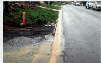
SOIL AND EROSION CONTROL WORKS
